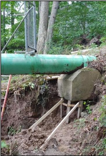
Sewer main crossing with temporary shoring of concrete abutment prior to new footing being placed.
